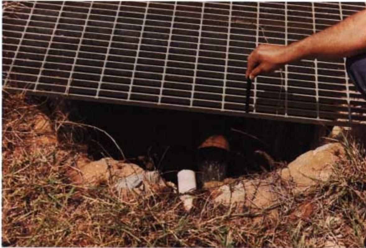
Figure 5. Reinforced sinkhole receiving plant waste water at the RCA del Caribe Facility. Waste water appears as clear water discharging from the rust colored pipe inside the sinkhole.
