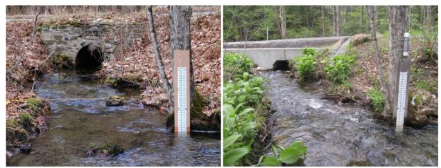
Figure 29. A culvert replacement downstream of a stream gage on Gulf Brook in Pepperell, MA caused enough of a channel change to necessitate a new rating curve.
