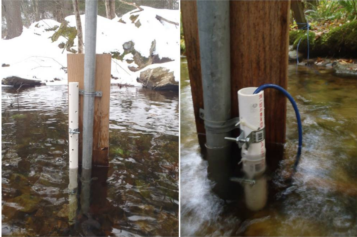
Figure 25. Non-vented (left) and vented (right) pressure transducers attached to staff gage board using conduit hangars.
