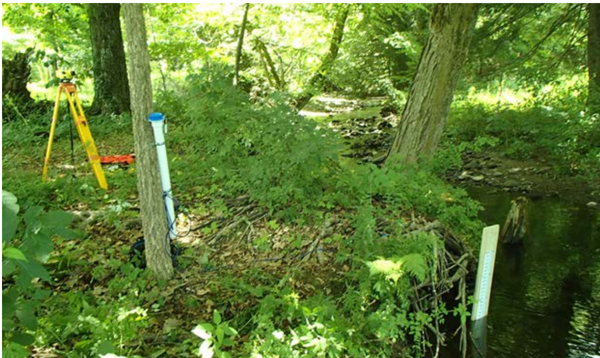
Figure 27. Vented transducer data logger installation. The transducer is attached to the tree with stainless steel conduit straps.
