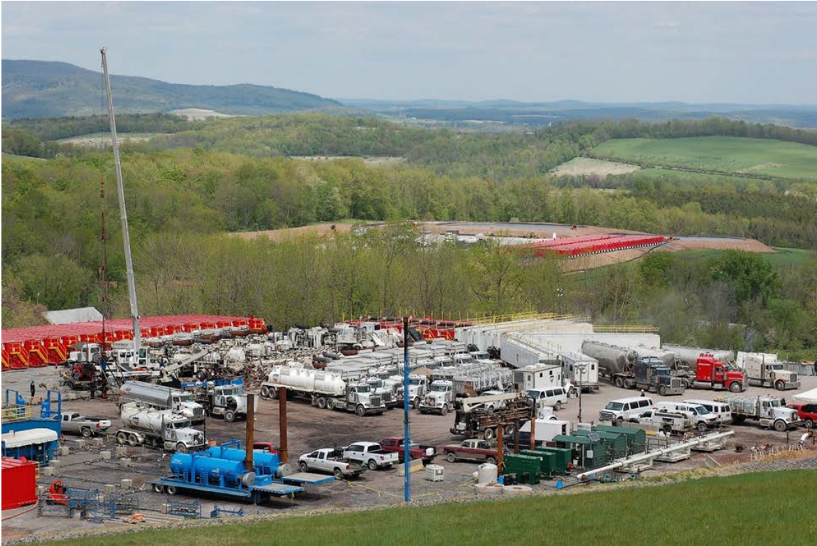
Figure 2-8. Hydraulic fracturing operation in Troy, PA.
