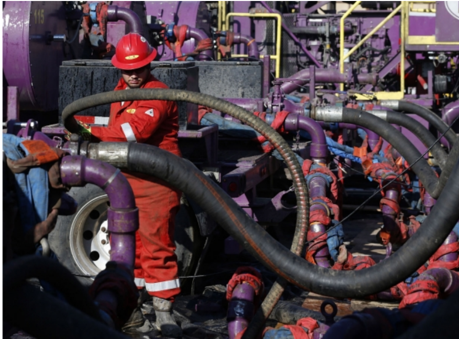
Figure 5-8. A worker adjusts hoses at a hydraulic fracturing site near Mead, Colorado.
