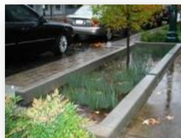
Figure 4. Street planters collect and absorb runoff. Source: EPA
