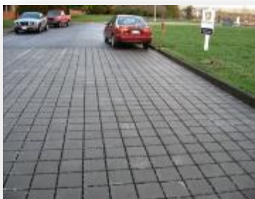
Figure 3. Permeable pavements reduce runoff. Source: EPA
