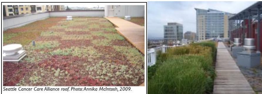
Figure 1. Examples of extensive (left) and intensive (right) green roof implementations. Images obtained from “Green roofs in Seattle: A survey of vegetated roofs and rooftop gardens”, which was prepared for the City of Seattle and the University of Washington Green Futures Lab by Annika McIntosh in August 2010 and can be located at http://www.seattle.gov/Documents/Departments/OSE/Green-Roofs-In-Seattle.pdf
