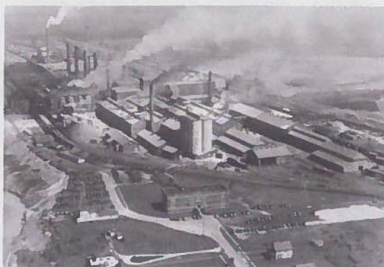
Diamond Shamrock chromate production plant, 1937, Painesville, Ohio
